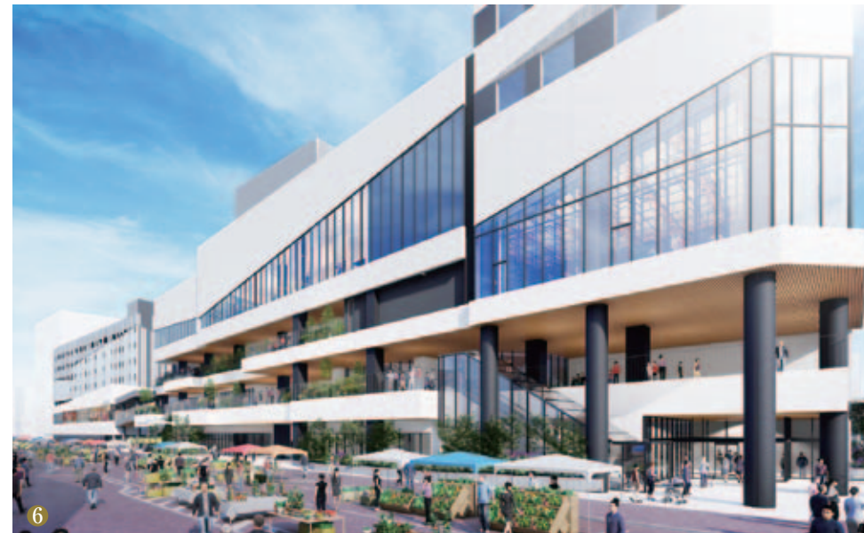
Image of the completed exchange and visitor attraction facility under construction in front of Fukushima Station.
