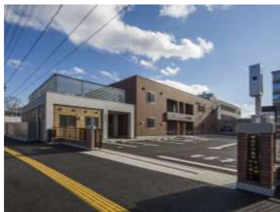
No. 2 [検査棟 (犬猫保護施設)]
